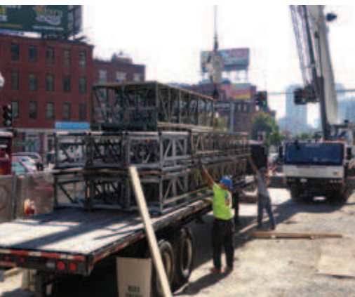
Marr Crane & Rigging provided installation and dismantling services for the Hydro Mobile units, seen here.
